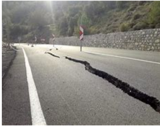
Figure 2.40: Cracks in a road
